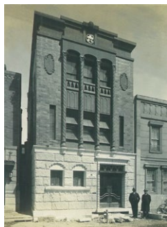
Head office at the time of the Company's founding
